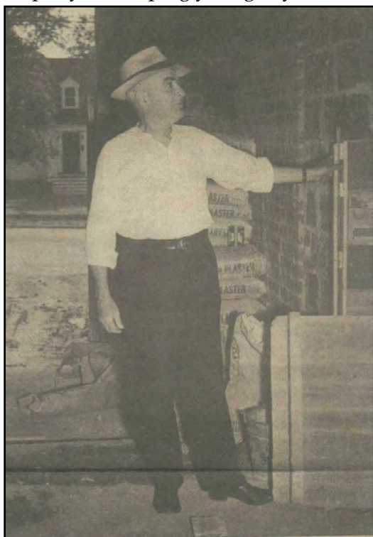
FATHER EDWARD V. MULLARKEY INSPECTS THE NEW SCHOOL UNDER CONSTRUCTION
